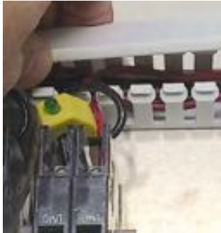
1) Remove wire raceway cover.
