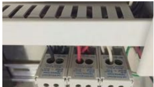
7) Replace the wire raceway cover.
