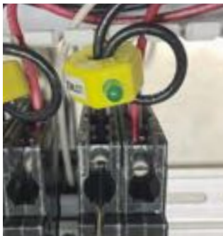
5) Secure the line side L1 & L2 wires to the top of the Breaker looping the L1 Wire through the LED Current Indicator.
