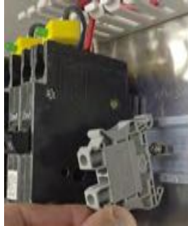
2) Snap the Terminal Block onto the DIN Rail.
