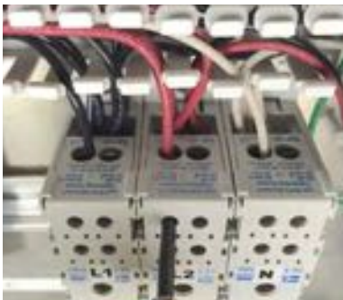
6) Secure line side L1, L2 & Neutral wires to the top of the Distribution Blocks labeled L1 & L2.
